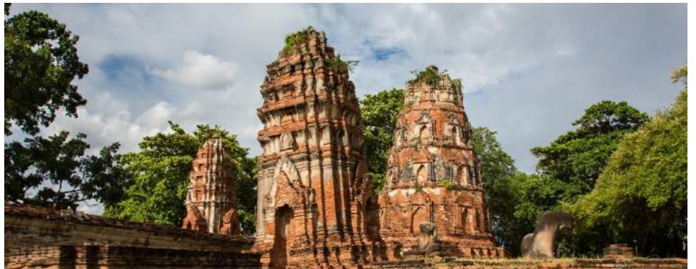
REMAINS OF WAT MAHATHAT, WHICH WAS BUILT OF LATERITE IN THE 14TH CENTURY AND RESTORED OR REPAIRED SEVERAL TIMES THROUGHOUT THE PERIOD.
